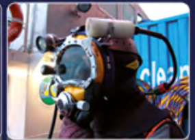
Diving Repair Works
